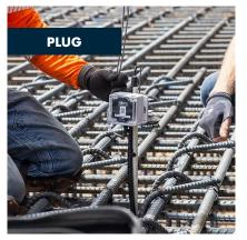
Plug the sensors into the transmitter node for wireless connectivity.
