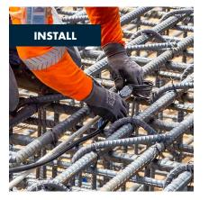
LumiCon sensors are easy to install. Simply secure the sensors to rebar with tie wraps.
